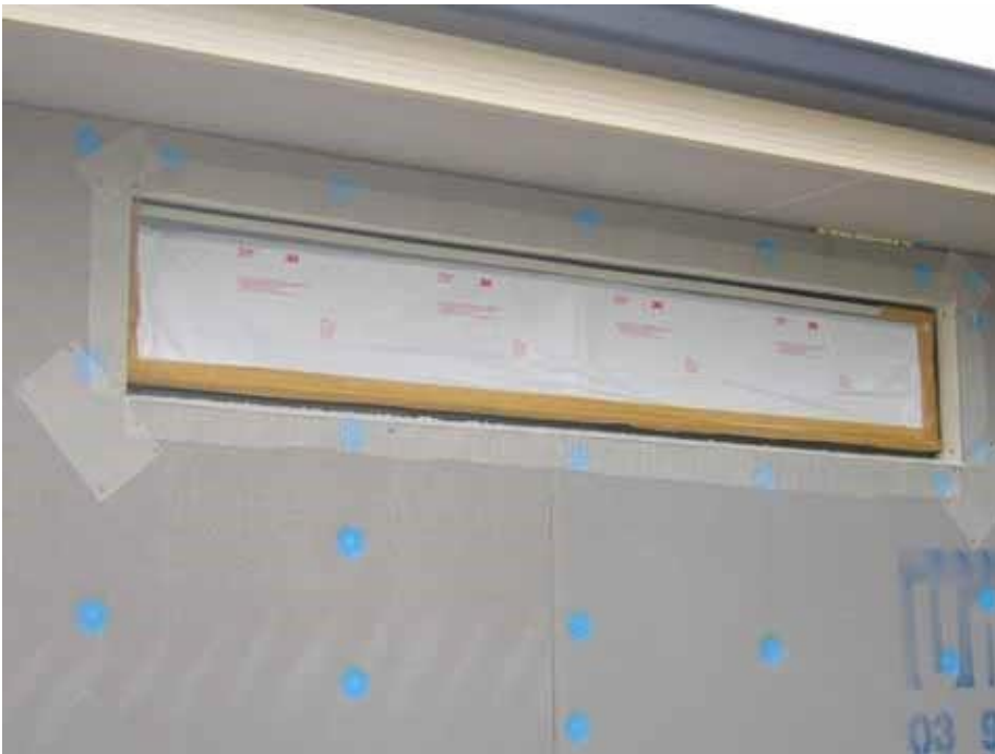
Fastener Positioning Details
