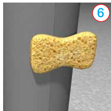
6 Sponge finish while the polymer render is touch wet, using sponge or polystyrene block
